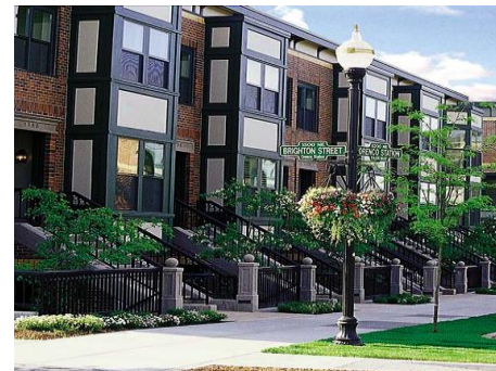
Buildings oriented to the street with windows along the front of the building reinforce natural surveillance of the street.
