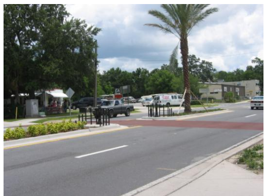
Trail street crossings should be clearly demarcated to increase driver visibility of trail users.
