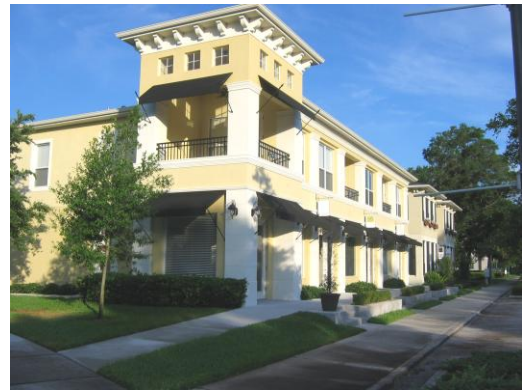
This mixed use development has dwelling units on the second floor and office space on the first.
