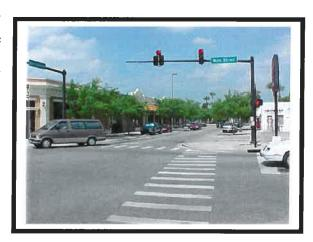
pedestrian signals on the west and north sides of the intersection. Only the west side, for north/south crossings, has high visibility markings on the pavement. Two additional intersections, Main Street/Adams Street and Main Street/Jefferson Street have curb cuts and high TBE Group, Inc.
